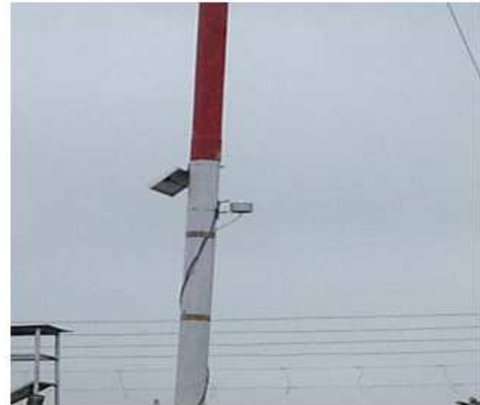
Fig.: 1- Snap shots of wind mast system at energy park, rgpv, bhopal, india
